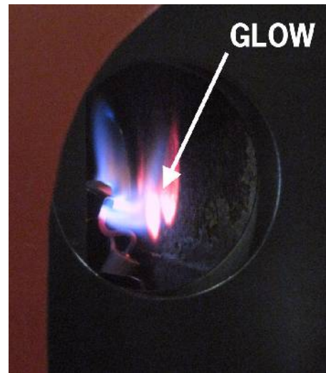
Illustration 5: Pilot Light Has Warmed Pad – Heater with Easy to See Heated Areas in Dim Light
